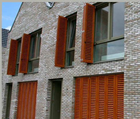
samenhang in gevels
